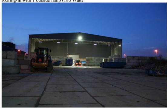
The existing garage (height 6,5 meters) was using 88 fluorescent lamps (36 Watt) and were providing 60 lux on the floor. They were replaced by 36 strips (50,5 Watt) and 2 spots (18 Watt). The result is >220 lux (general) and container repair unit 325 lux.
