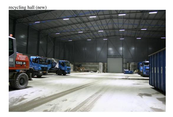
The lamps are at a height of 12 meters and the distance between the frames is 10 meters. The distance between the lamps, on the frames, is 5,5 meters and have been divided as 50,5 Watt -4 times 101 Watt -50,5 Watt . The amount of lux on the floor is 70-180 lux. To get 200 lux on the floor we need twice as much strips (101 and 202 Watt) but the principal is very satisfied (never had so much light) so pity they did not do.
